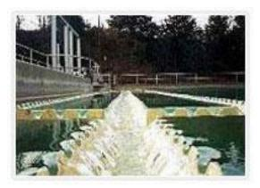
The collection of water in weirs in the clarification basin after additional detention time has allowed more suspended particles to settle.
