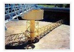
An empty East Plant sedimentation basin shows large sweeps and blow-down structures used to collect and dispel settled solids.
